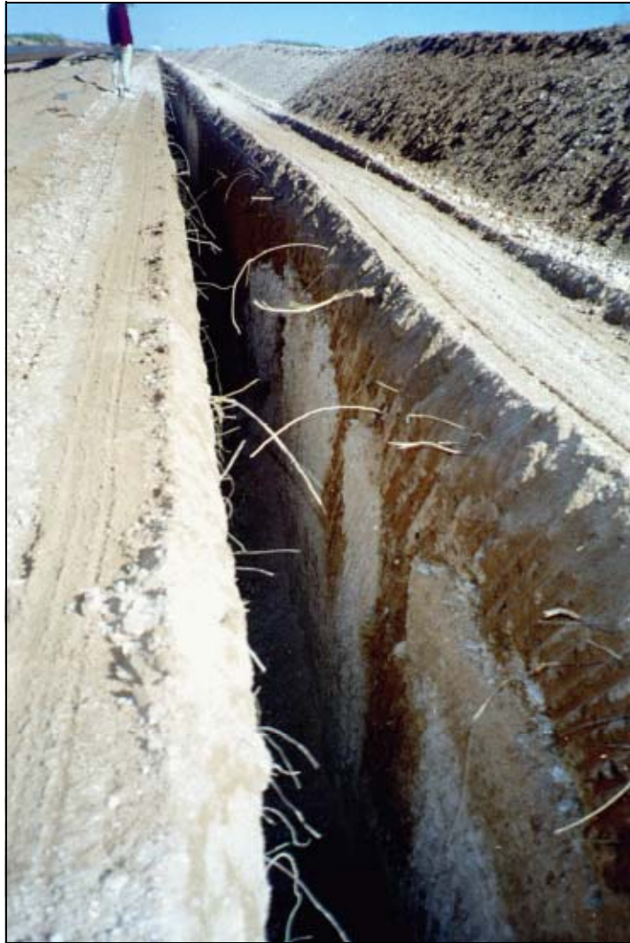
Figure 3 Typical pipes observed in Section One of the transect on the Lower La Mesa surface (New Mexico).
